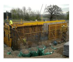
This project covers 5 water treatment tanks, 100 metres long by 50 metres wide and 5 metres high. Each tank had several complex baffle walls and suspended channels incorporated into it. The customer chose to purchase for the project in order to meet their ongoing needs.
