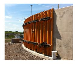
This project took 34 hinged corners for the photographed wall, as well as this, a 6 metre high trash screen was constructed along with a culvert using enkoflex horizontal formwork with Orma used for the walls
