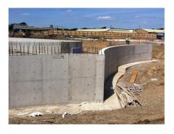
Both Orma and Bira combined together to allow this project to pour awkward shapes in one complete pour..... allowing the project to flow uninterrupted by complex curves turning into straights. The finish was left on view on the outside, so the quality finish was needed. As you can see the excellent concrete results allowed the contractor to finish the job happily ahead of schedule, without the need for much rubbing up at all.
