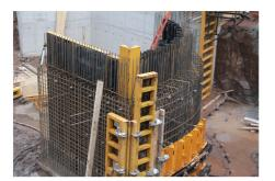
This wall changed thickness from 450 mil to 600 mil at the angled corner and proved quite a challenging design which Orma and Bira combined using hinged corners was the only solution for this radius stairwell on the site.
