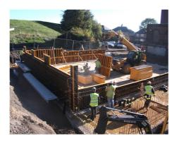
Poured in one as a 60 metre long stretch in total to eliminate any joints for this watertight tank was the sites requirement for this project -this request was made on the Wednesday and our operations team prepared the delivery for the Friday helping the contractor to jump one week ahead of programme.
