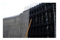
The wall height of 6.6 metres was achieved using BIRA panels stacked – with the grout check feature stopping any grout loss in the horizontal joint an F4 finish was achieved. This was the only system avalaible which ticked all the boxes for the site who's craneage and site access were a challange for the site team to say the least.
