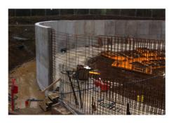
This repeat user of BIRA had to construct a 4.5 metre high tank, utilising their existing own BIRA with additional material supplied by Adapt Formwork, 40 metres diameter constructed in 4 pours.
