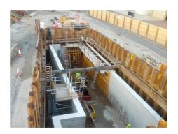
This sewerage works as part of the Yorkshire Water AMP 5 programme saw this 5 metre high CSO chamber along with a 20 metre deep pit constructed in 5 lifts in the height.
