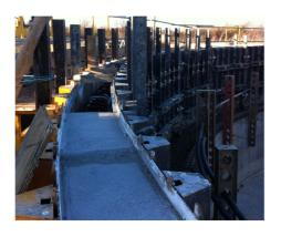
BIRA was radiused in 2 lifts to form this Sludge Digestor Tank as part of the AMP 5 Framework. Due to the 1100 wall thickness timber infills were used in between the BIRA to form the shape. Quality F4 finishes every time using BIRA.
